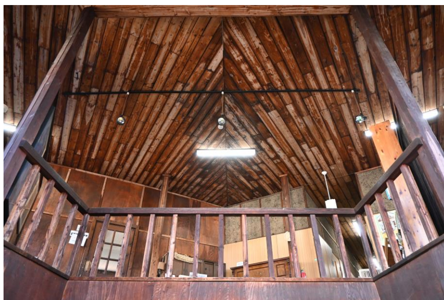
0 9 2階ロビー天井
